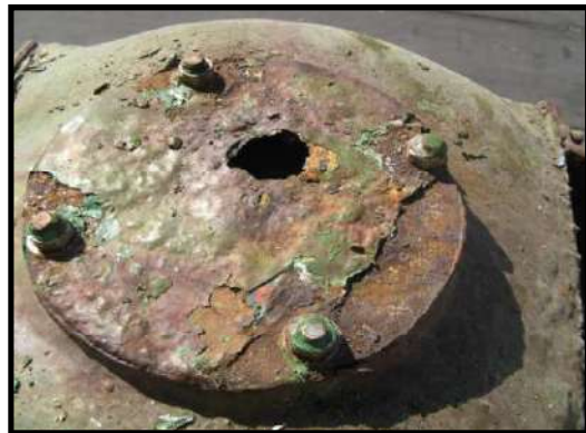
Defective Air Vent
