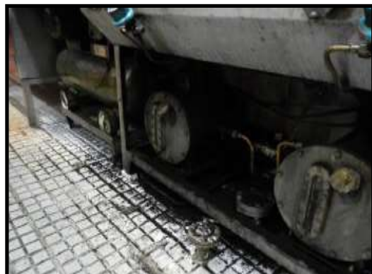
Unsafe ignition process/fire hazard for diesel fired work in galley
