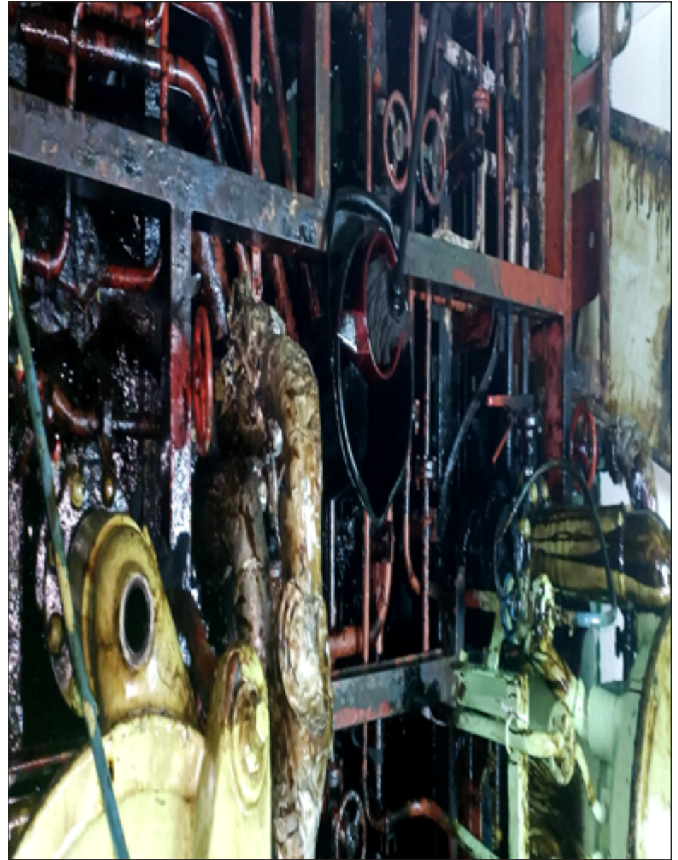
Engine room tank top full of water and over all cleaning condition not as required [Insufficient]
