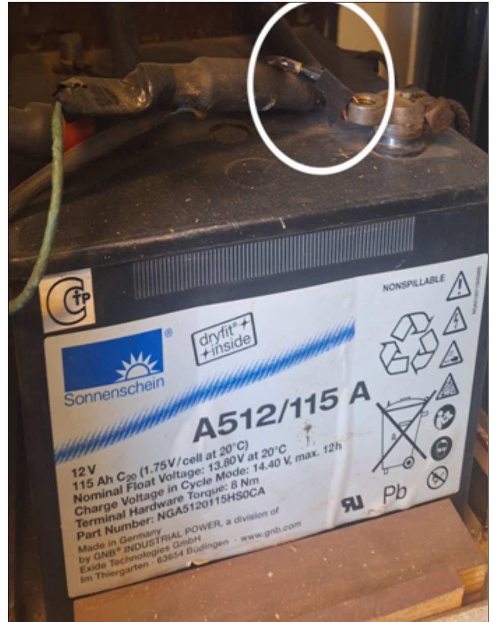
One Set of Battery not Properly Maintained for Start of Emergency Diesel Generator. Weak Cable Connection. [not properly maintained]
