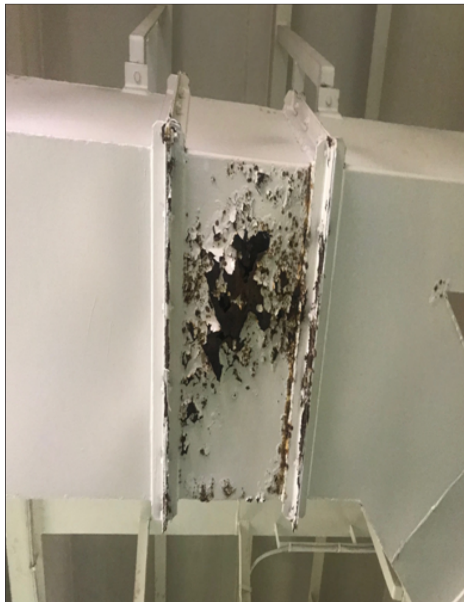
Steering gear room intermediate inlet ducting just above telephone exchange area found completely corroded and wasted. [Not as required]
