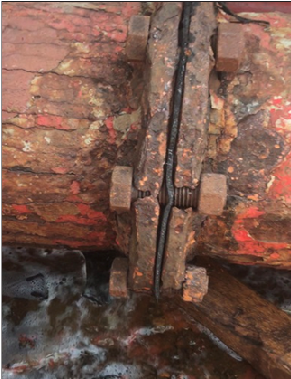
Deck main fire hardly corroded and holed and leaky [Not as required]
