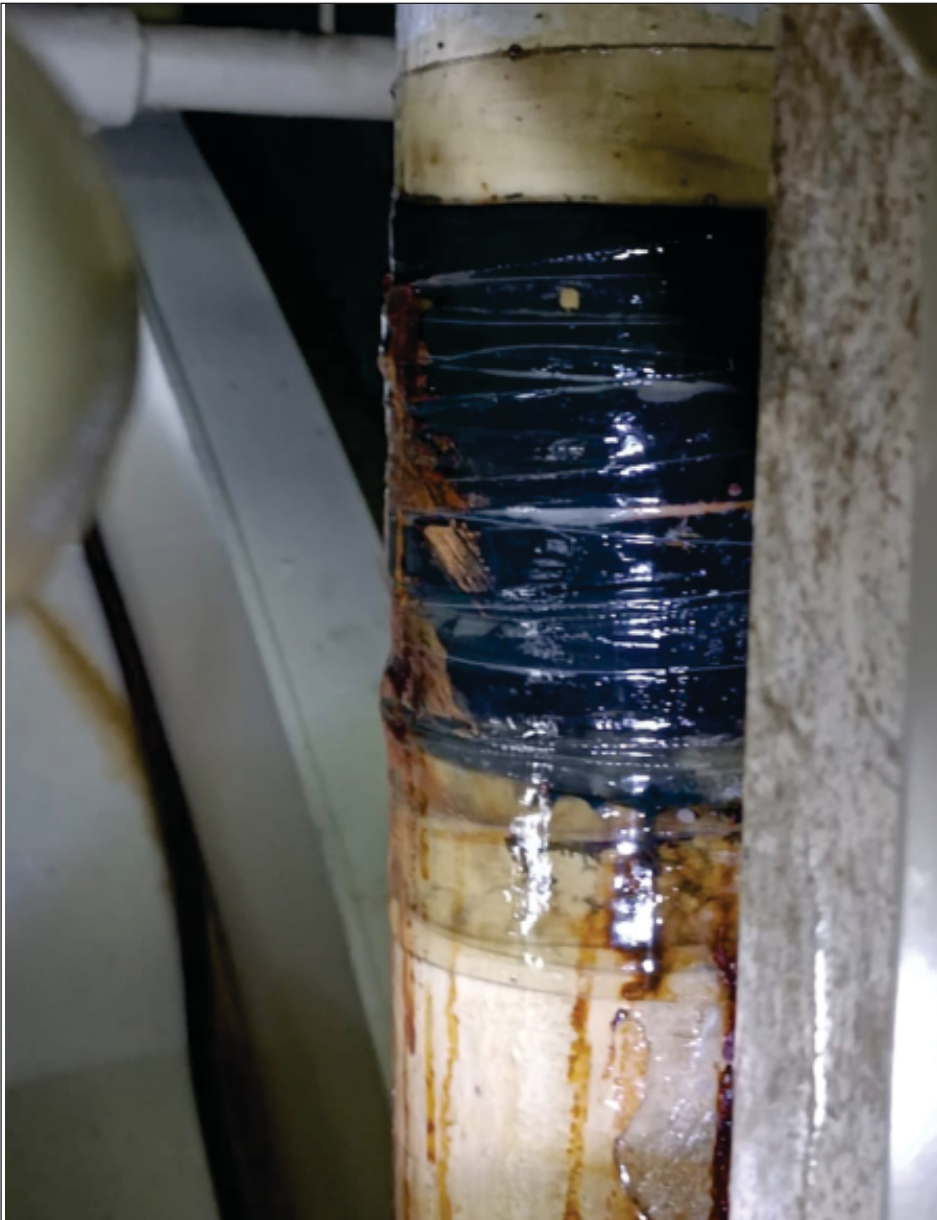
Galley Drain Overboard line found leaking. [not properly maintained]
