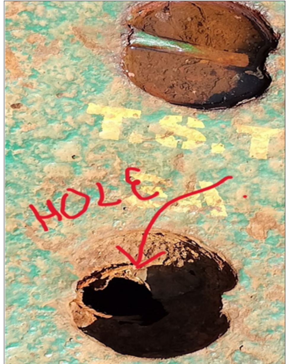
Manhole cover TST 3A holed, rubber damaged, missing nuts [cracked]
